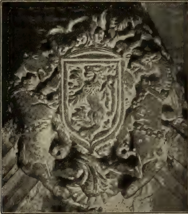
FIG. 2.—Carved Boss in Vaulting of Aisle of Car Fergus.
